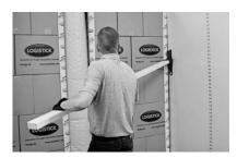
**Removing Tape Remnants:** Use a cloth, and if needed, a scraper and a citrus based adhesive remover to clean any remaining tape residue from the trailer walls.
